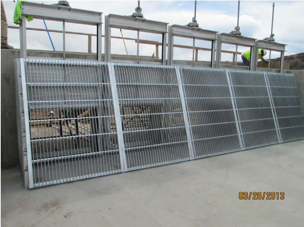
**Inlet Structure with New Gates and Trash rack**
