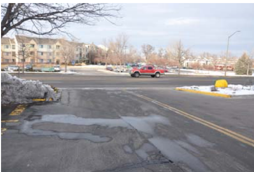
Main Driveway from Elizabeth
