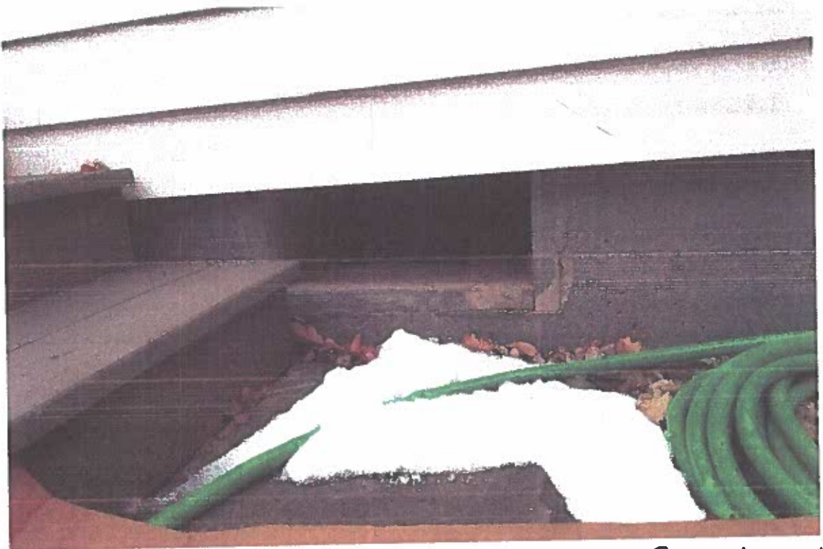
EAST SIDE VENT #2
